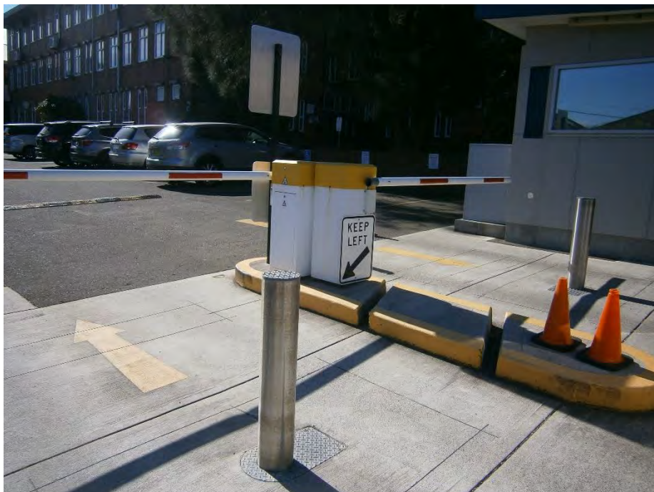
Security rising bollards and boom gates at entry/exit driveway of Car Park 1
